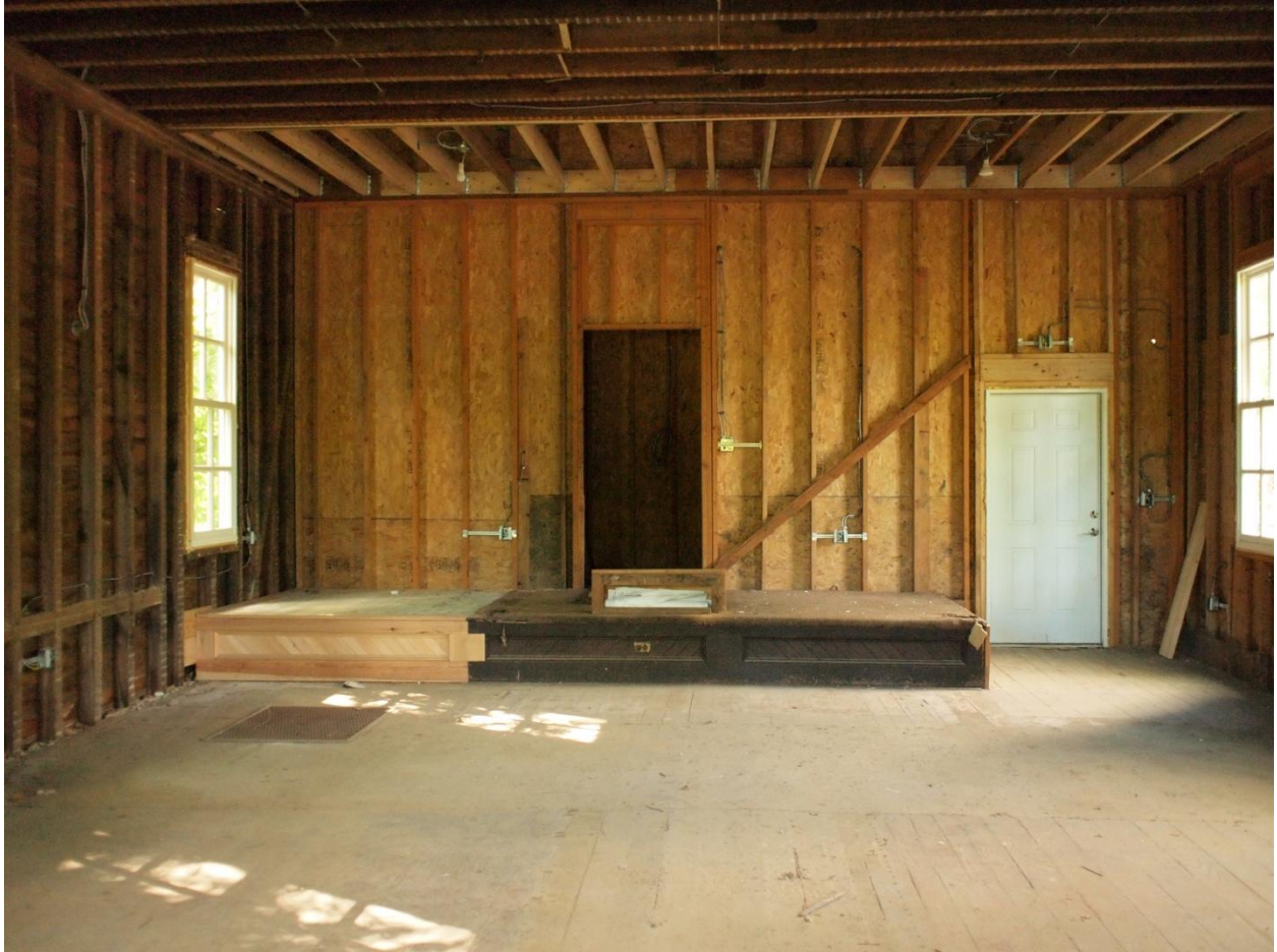
Interior renovation is underway.
