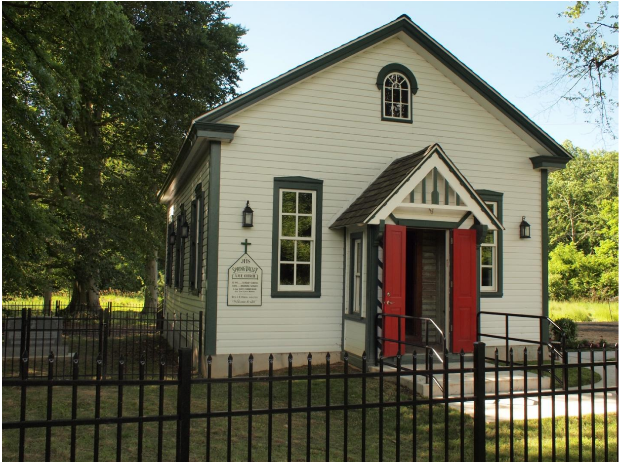
Renovated church exterior.
