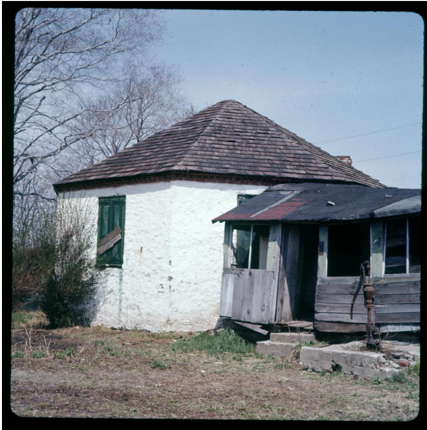
The Octagonal Schoolhouse, side April 18, 1959
