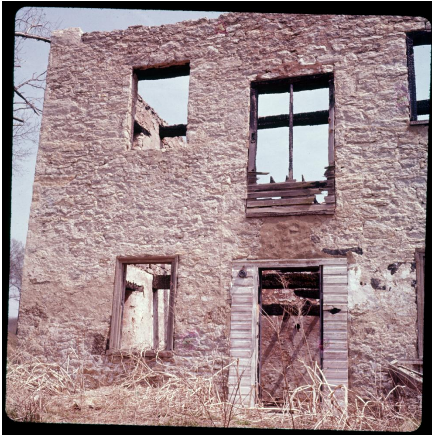
Harvey Mill Ruins, close April 18, 1959, Route 1
