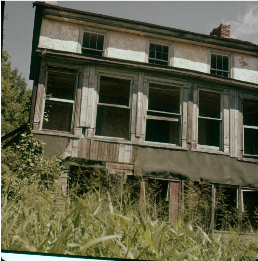
Roche's House ruins, from front June 12, 1959, Smithbridge Road
