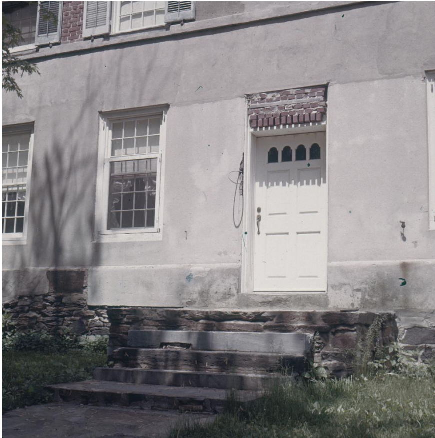
Row houses, closeup May 14, 1959, Dilworthtown
