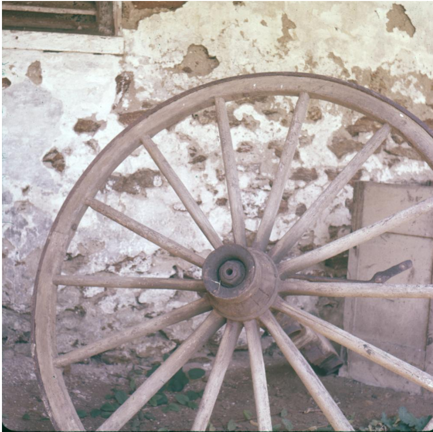
Roche's House ruins, close, front porch with wagon wheel June 12, 1959, Smithbridge Road
